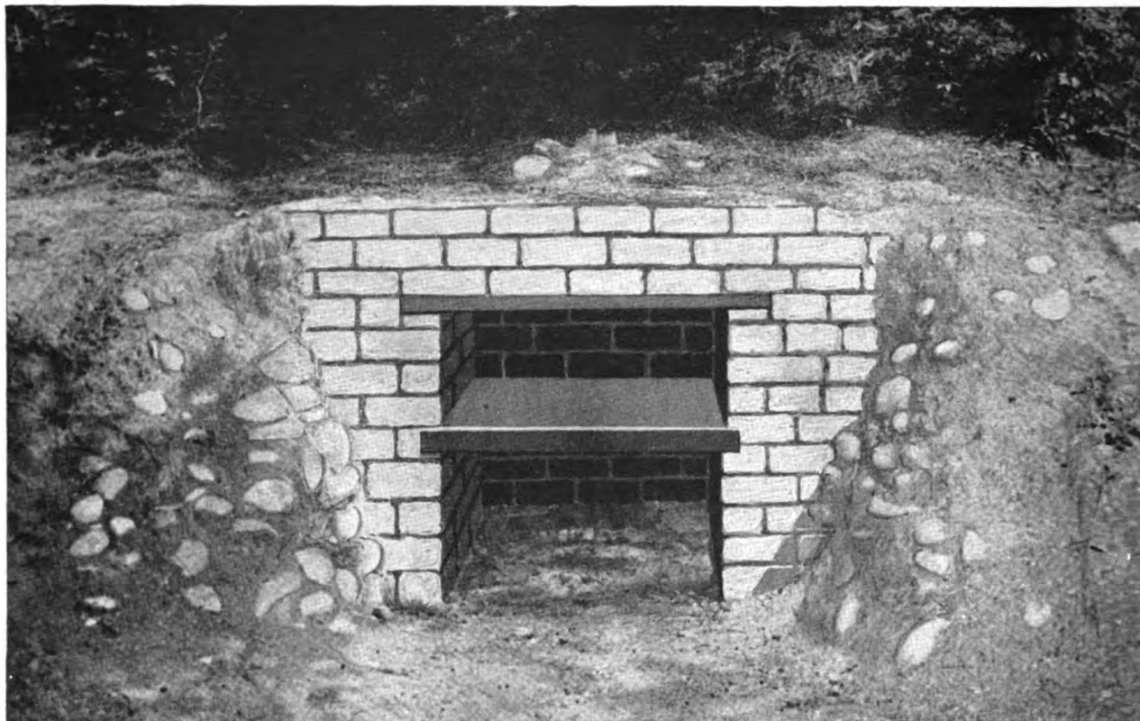
Figure 76. Improvised earth oven with firing and baking chambers.
